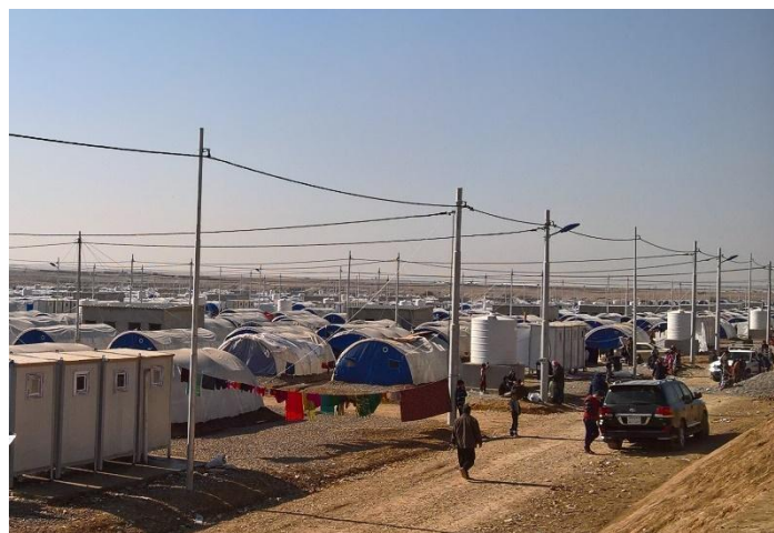
Figure 2: Electricity supply in Kirkuk camp (source: www.reach-initiative.org )
