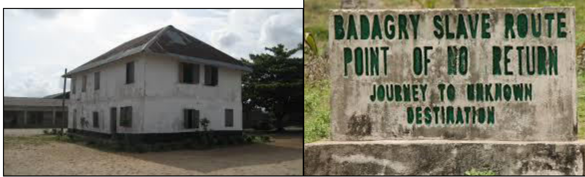
Fig. 2. First storey building in Nigeria
