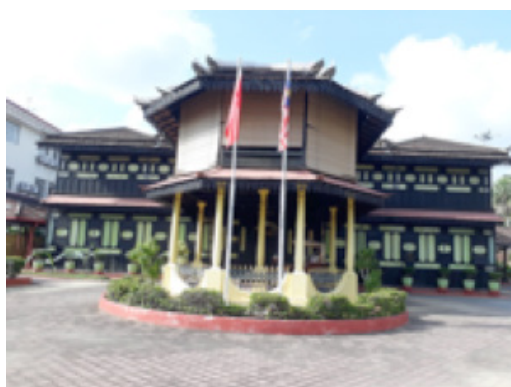
FIGURE 5a. The building of the Kelantan Royal Traditions and Customs Museum (the Jahar Palace, Kelantan) Source: Author (2018)
